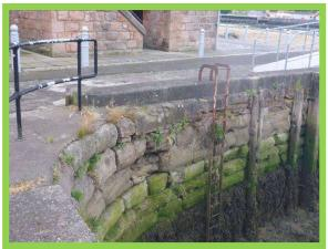
Masonry quay walls in dock area in fair overall condition with some open joints, cracks and abrasion (/0801C03)
