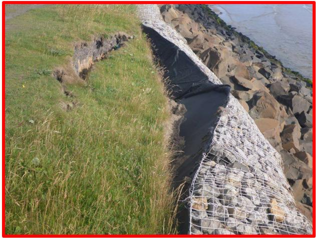
Rotational failure of one section of gabion basket caused by cliff slumping – requires maintenance (/4001C01) – <u>locally</u> very poor
