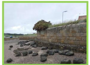
2801/C02 Masonry wall with concrete and cobble toe apron. Little change.
