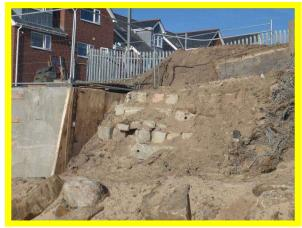
*Tie-in section of wall at failing gabions (/4201C04)*
