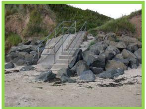
2601/C09 2018 low beach level and 2601/c09 higher beach levels to toe of steps. undermining.
