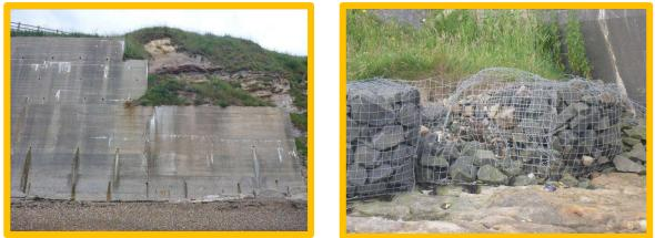
One of three notable vertical cracks in the sea *Break-up of gabion baskets (/4401C19)* wall *(/4401C17)*
