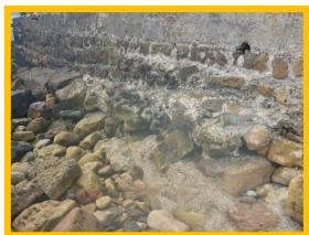
Heavily abraded Beadnell Harbour wall (outer face of eastern wall) (1701C47)
