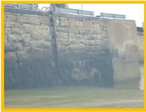
Scour holes and possible undermining around low Heavily abraded outer face 1701/C14 water mark – 2018 1701/C14
