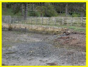
2801/C10 Local undercutting of concrete toe to 2801/C10, slight damage to downstream end. repaired section
