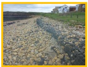
Damage to gabion basket wall at (Lady's Hole) gabion wall – partially submerged to high sediment levels. (/1701C40)
