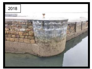
Undermining of Beadnell Harbour wall (inner face of southern wall) 2018 (1701C51)
