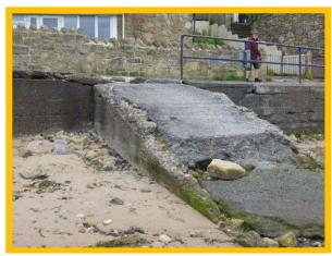
Access ramp to Little Shore Wave Basin in poor condition in 2018 (/3001C10)
