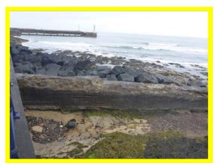
Abraded but functional stub groyne (and rock armour) on seaward face of South Pier (/3101C02)
