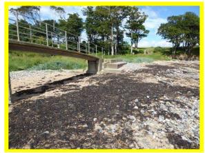
2501/C01 Undermining of concrete at southern bridge abutment. Higher beach levels since 2018.
