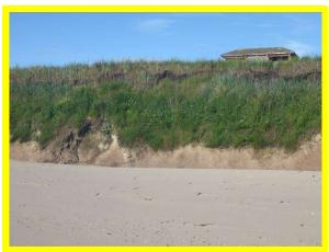
Erosion of cliffs at terminal end of rock revetment (/3901C03)
