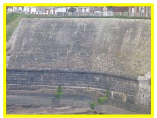
Seawall with upper brickwork retaining wall (/4401C15)
