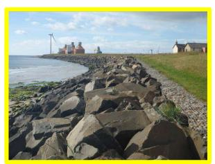
Rock revetment with gabion baskets at rear (/4001C01)
