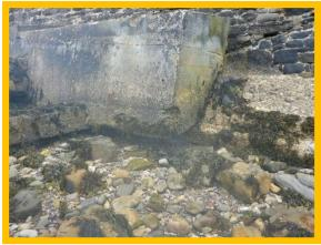
Undermining of seawall at Beadnell North (Nacker's Hole) (/1701C36)
