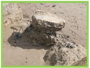
Heavily abraded concrete anti-tank block with exposed rebar (/2901C02)
