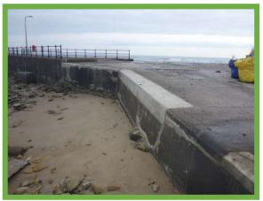
Repairs return sea wall along Bay View to good overall condition in 2020 (/3001C10)
