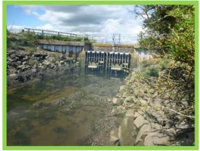
1401C18 – Good condition sluice at Ross Low channel
