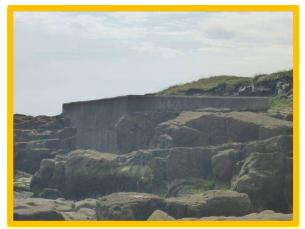
Seawall with undermining and outflanking (/3501C08)
