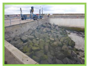
Rock armour in good condition, concrete sea wall behind is heavily abraded. 1701/C10
