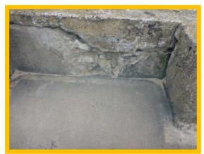
Damage to splash wall (1701C47)
