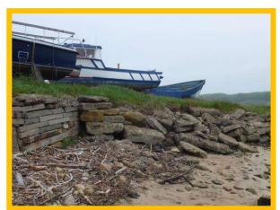
Partially collapsed section of Wansbeck Boat Club retaining wall (/3801C02)
