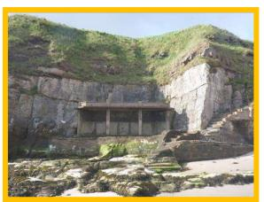
Concrete pavilion structure in fair/poor condition, missing brickwork from fronting wall (/0701C02)
