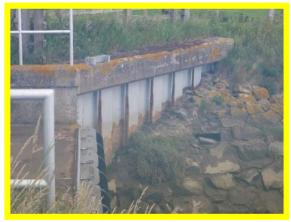
1401C17 – Corrosion and marine growth evident on sheet piles at Ross Low sluice
