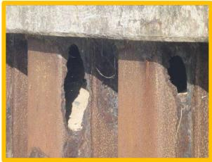
Voids in steel sheet pile end to promenade (/4201C08)
