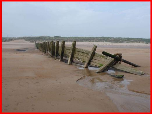
Failed seaward end of southern groyne in 2018 when beach levels were low (/4301C01) – not so visible in 2020 due to high beach levels partly burying the collapsed section – locally very poor
