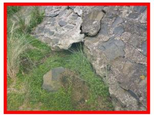
1401C27 – Localised section to the north of mortared revetment failed. Extensive cracking and washout of material.
