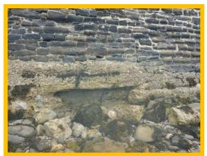
Loss of mortar, damage to blockwork of seawall and abraded concrete toe at Beadnell North (Nacker's Hole) (/1701C36)
