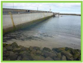
Concrete encasement and cope repair to inner face of north breakwater. 1701/C09
