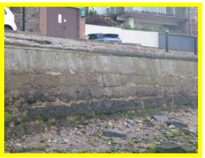
Local failed section of river slope revetment/wall Local damage to wall coping (/0801C07) (/0801C07)
