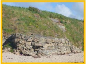
Short seawall with active breaking-up apron (/0701C07)
