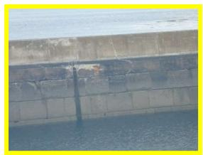
1701/C21 Some spalling visible on concrete cope.
