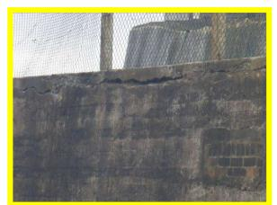
Cracks in private seawall around Pan Point (/3101C04)
