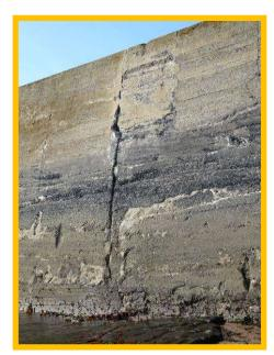
2201C03 Crack in north pier. Minor spalling
