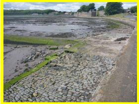
Local failed section of slipway over foreshore outfall (/0801C07)
