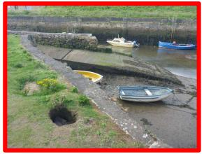
Undermining at toe on inner face of boat ramp (/4401C05) – locally very poor
