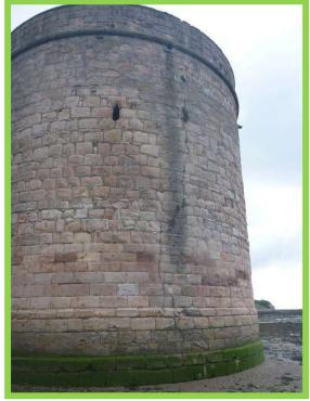
Vertical crack in wall at roundhead (/0801C06)
