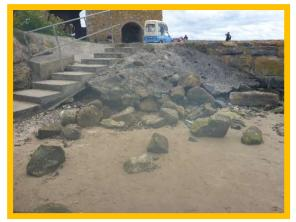
Undermining and partial collapse of grouted stone revetment adjacent access steps. (/1701C53)
