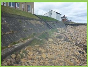
Concrete revetment in good condition, evidence of grout repairs at southern end (/1701C42)
