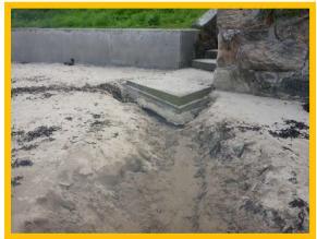
1701/C16 Undercutting of toe of steps, adjacent wall remains in good condition.
