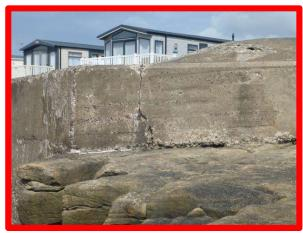
Second length of seawall with undermining and outflanking (/3501C10)
