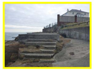
Heavily abraded access steps to Pan Point (/3101C02)
