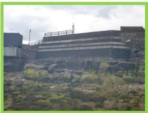
No significant damage - minor abrasion noted to the concrete toe (170104)
