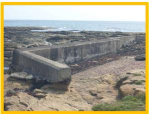
Seawall with undermining and outflanking (/3501C08)
