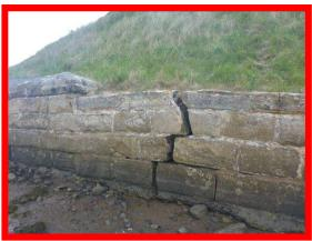
Displaced blockwork in wall at Church Hill Cracked section of wall at Church Hill (/2801C13) (/2801C13)
