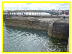
Poor condition at junction of South Pier and South Jetty (seaward face) in early 2018 (/3101C01)
