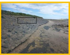
1401C29 – Depleted beach levels believed to be causing washout of material resulting large cracks opening.
