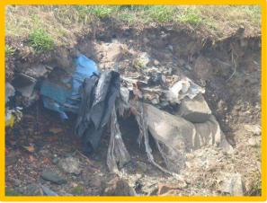
Refuse buried in eroding coastal slope above seawall (/3501C08)
