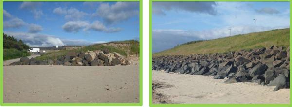
Reinstated and improved rock revetment protecting slipway (/3901C05)
