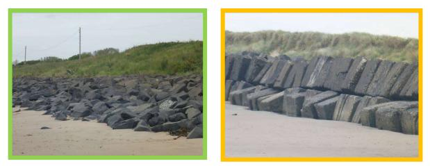
Wide rock revetment in good condition Rotational displacement at southern end of (/3201C03) concrete block revetment (/3201C04) Immediately south of this revetment is an outfall in poor (but draining) condition. It is clearly evident that
