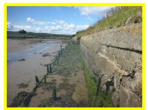
1401C14 – Concrete wall in fair condition. Timber toe erosion protection in poor condition.
