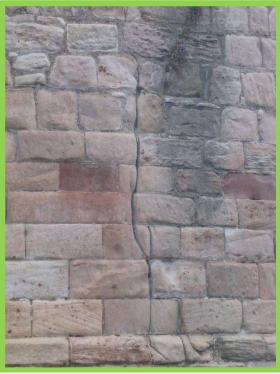
Vertical crack in wall at roundhead (/0801C06)
