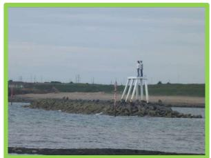
Detached breakwater in central Newbiggin Bay remains in very good condition with salient/tombolo developed in lee (/3601C15)
