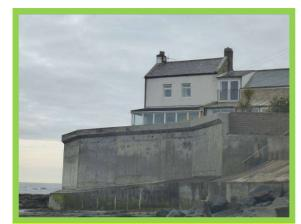
Substantial seawall in overall good condition (/3101C07)
