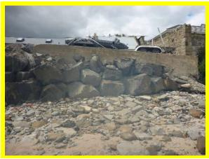
Concrete cast onto the crest of the revetment to provde flat storage area (/1701/C32)
